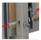
Clevis pin, spacer, and 'R' clip removal
